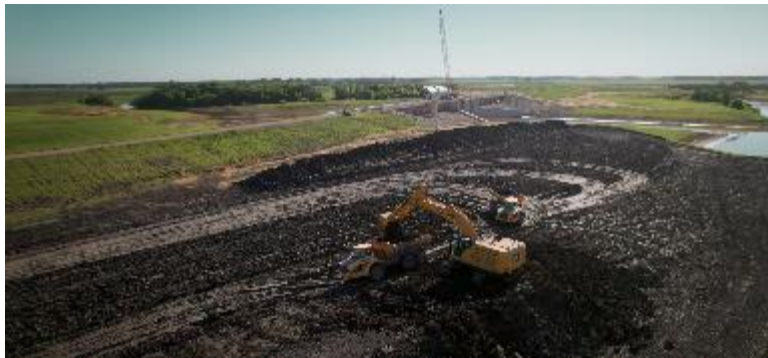
Reach 2B – 37% Completed
