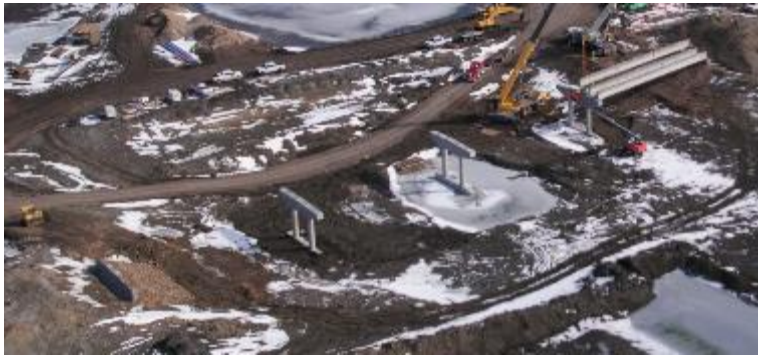
County Road - Substructures
