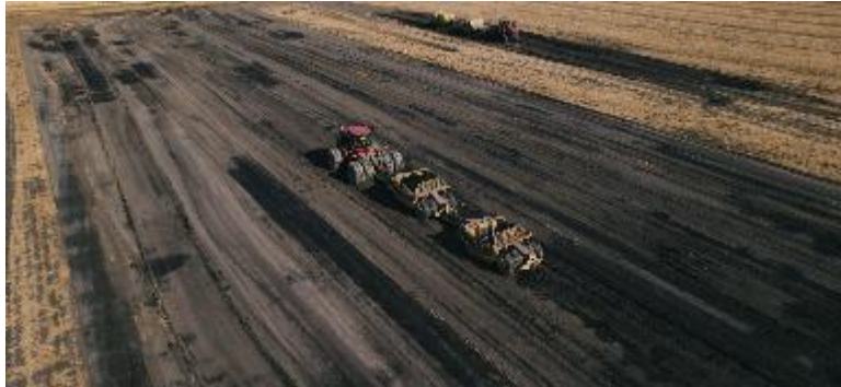
Reach 1A – 100% Completed
