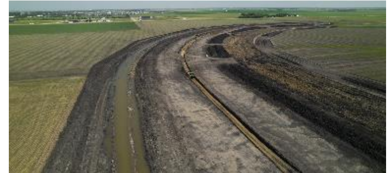
Reach 2A – 76% Completed
