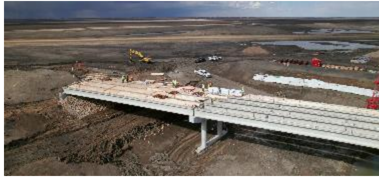
County Road - Deck Forming
