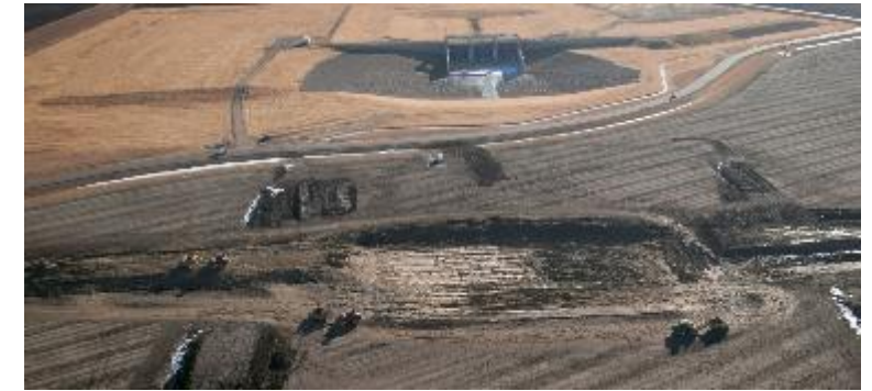
County Road - Preload
