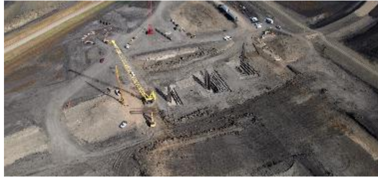
County Road - Piling
