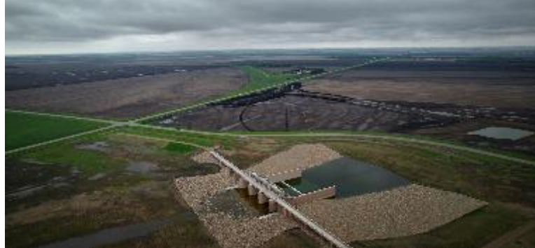
Reach 1B – 29% Completed
