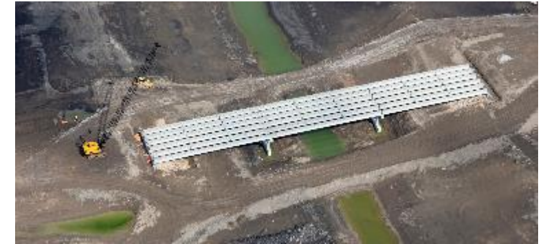
County Road - Girders
